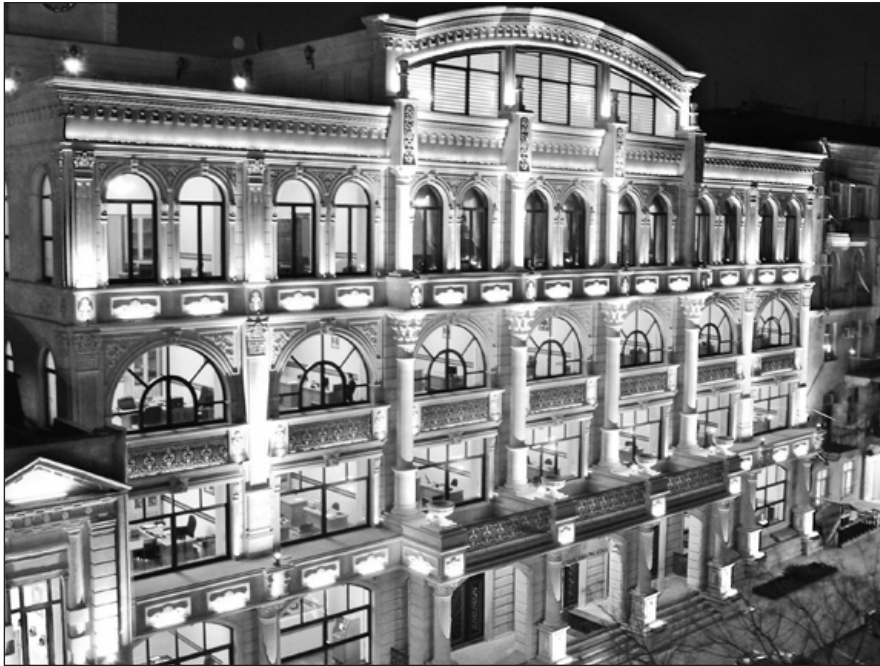
New building housing the Azerbaijan Chamber of Accounts
